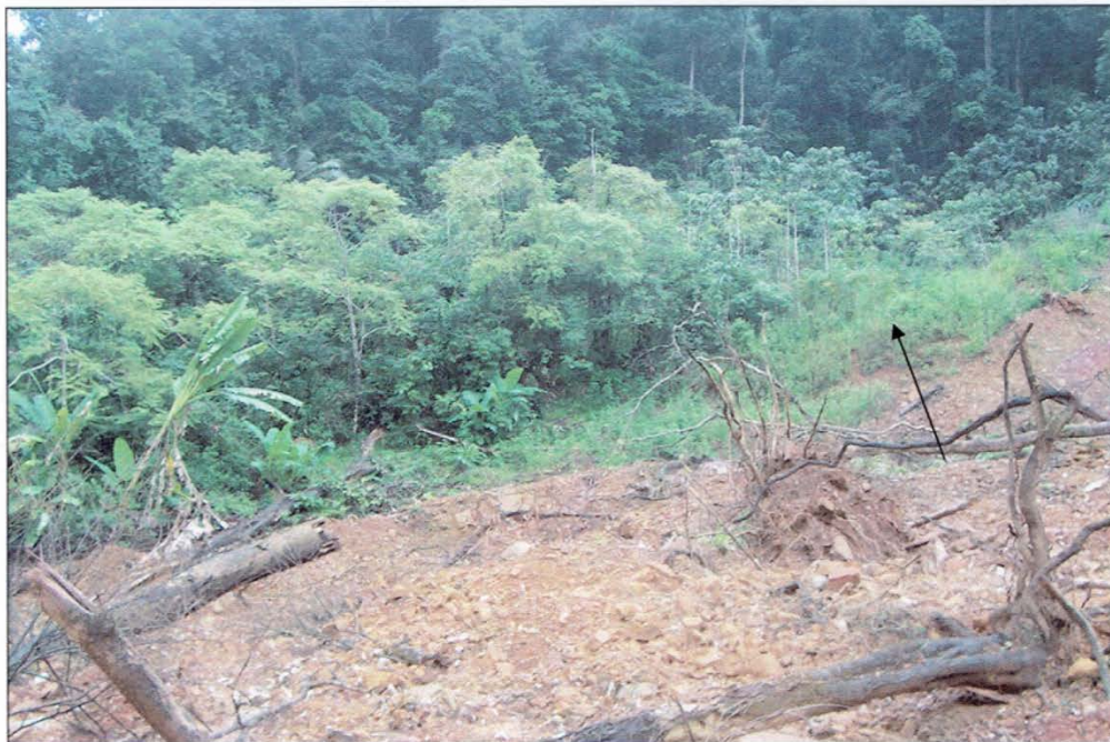
Photo 8: Right flank of the slide in the zone of depletion of the Hadgeri landslide. Old slide scarp is also seen.
